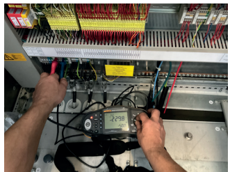
Resistance measurement
